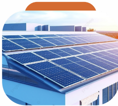
Solar Rooftop Solutions
